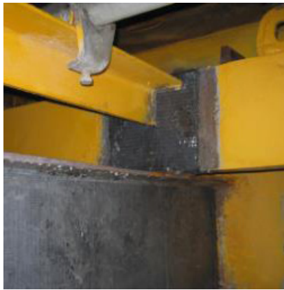
Walkway beams after repair
