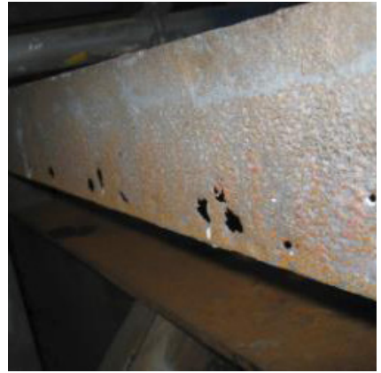
Walkway beams before repair
