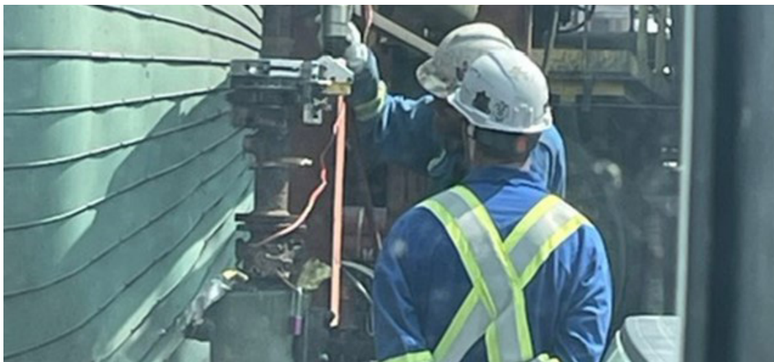
Technicians completing a Quickflange™ installation in a confined space with no hot work required
