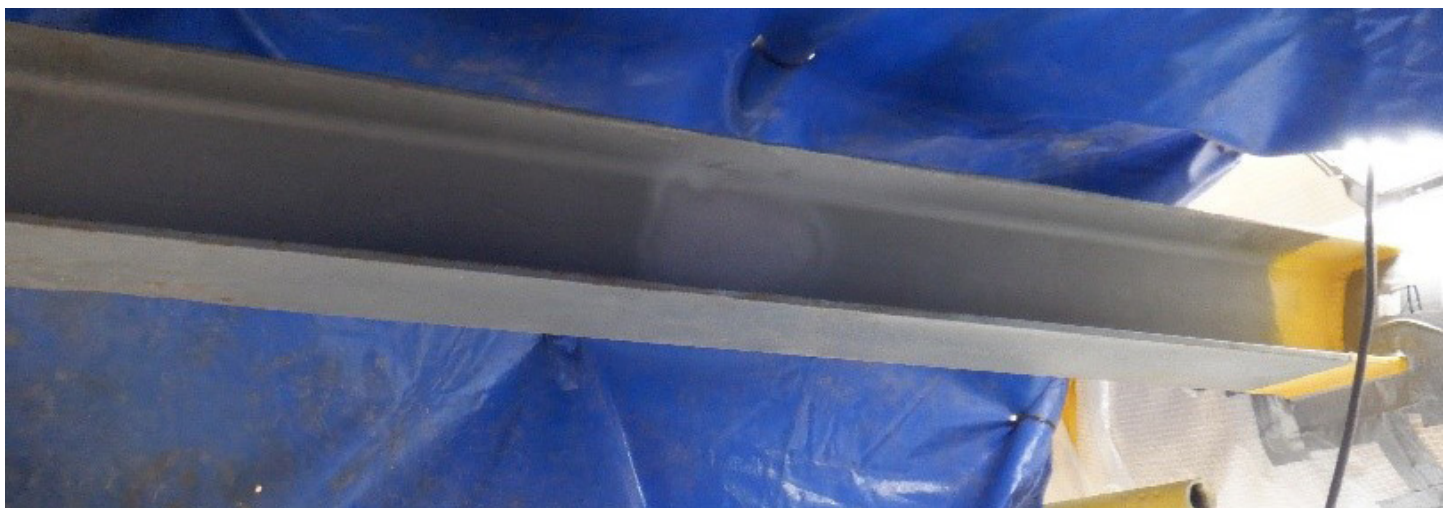
Beam after surface preparation, ready for composite repair.
