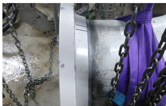
Completed Quickflange™ installation.
