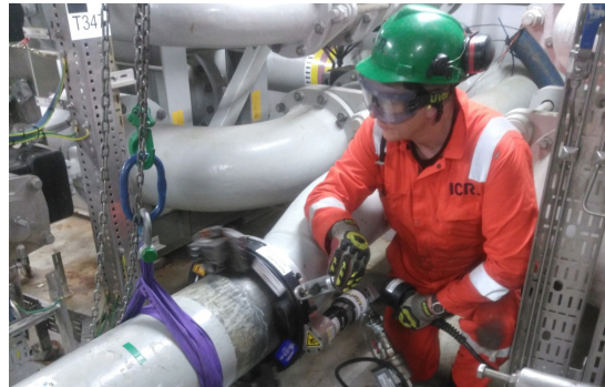
Cutting the pipe using orbital cutting equipment.
