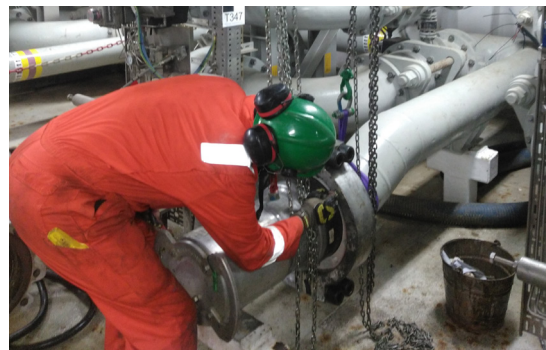
Installing the Quickflange™ connector using our installation tooling.
