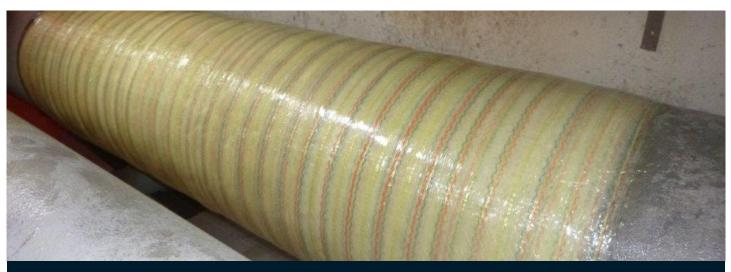
Composite repair carried out by ICR to reinstate integrity, with pipework remaining in-service at all stages of work
