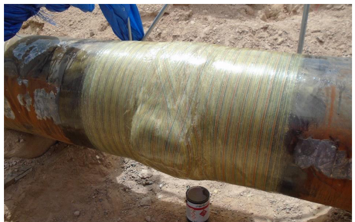
Layers being built up over the full length of the repair
