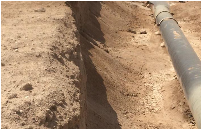
Excavated ground revealing buried pipework
