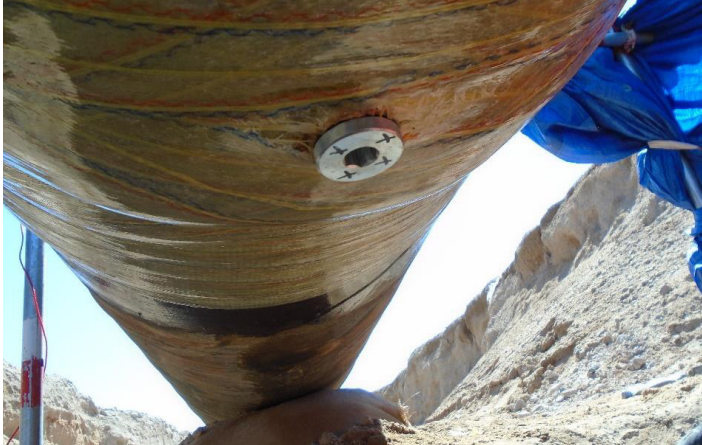
View of threaded nut secured in the layers
