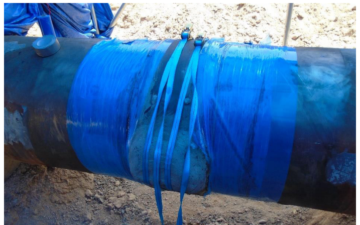
Sump held in place using ratchet straps and either side secured to the pipe with a composite repair
