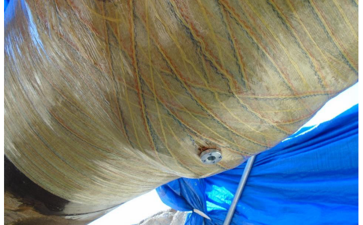
All layers applied and cured surrounding the nut
