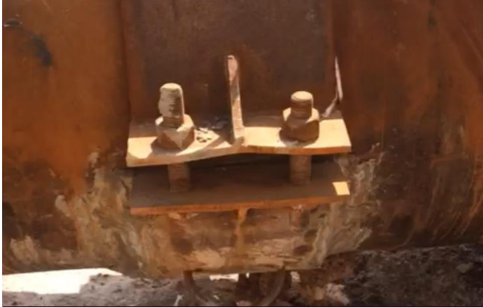
Clamp requiring profiling using Technoseal FP
