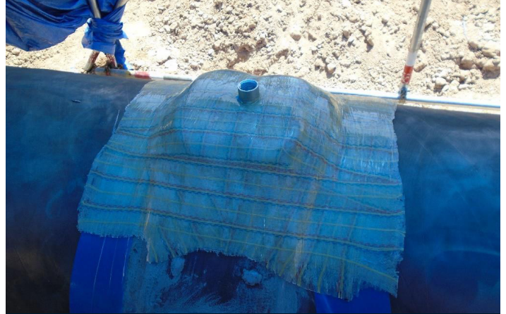
Composite sump formed at the top of pipe ready to be manoeuvred to the underside of the pipework
