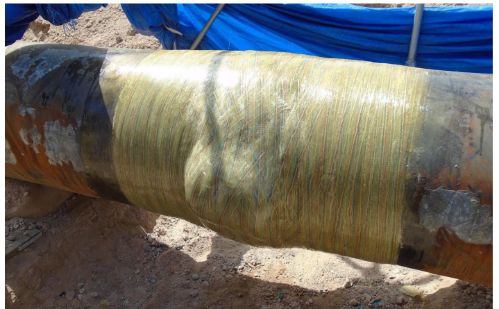
Completed repair encapsulating the clamp and leaking bolt hole
