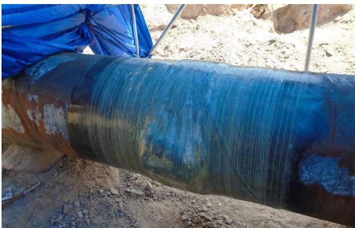
Once both sides of the sump had cured and held in place, layers were applied over the middle
