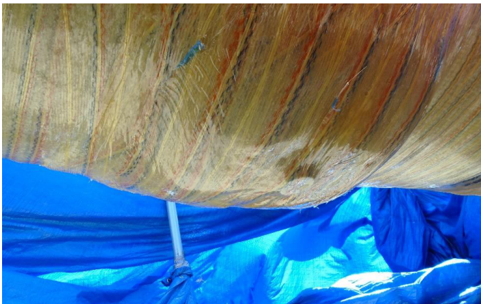
Threaded bolt fitted to nut to secure diesel in the sump. Cloth applied over the top of the bolt
