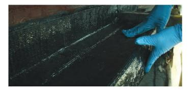
Our Technowrap SRS™ (Structural Rehabilitation System) utilises the unique features of carbon fibre technology intended for structural strengthening applications. It is less than one-quarter the weight of steel, which makes it 4 times as stiff on a weight to weight basis. It is approximately twice as strong in tension and it has a better fatigue performance than steel, aluminium or titanium.
