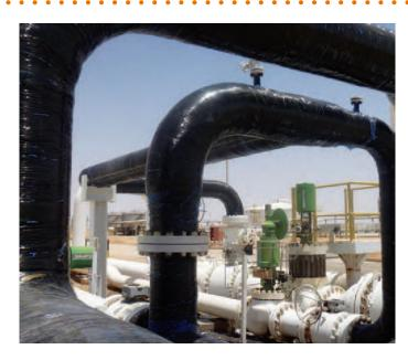
Technowrap H.P. PRS™ (High Pressure Pipline Repair System) has been designed for use on land. The system's intended application is for large diameters of pipe work, such as a 36 inch pipe operating at 50 bar pressure, and is ideally suited to the Middle East market. The uni-directional carbon based cloth applied with our epoxy resin system results in a fast application time.
