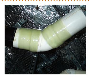
Technowrap Potable™ is a design engineered glass-based repair system specifically designed and certified for potable water applications and can be used on all pipe work components. It consists of a glass fibre reinforcement encased in an epoxy resin which has been specifically formulated for use in drinking water applications. The repair system has been successfully tested to BS 6920, confirming its suitability for potable water applications.
