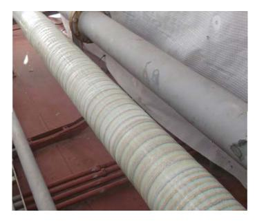
Technowrap™ Glycol is an original product from the innovative Technowrap composite repair product line. The multidirectional glass cloth used in conjunction with our specialised formulated epoxy resin system is developed for use for the repair of piping and vessels containing up to 100% glycol. Once applied Technowrap Glycol can seal through wall defects and re-instate the structural integrity of the defective pipe section.
