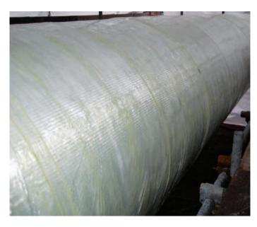
Technowrap PRS™ (Pipeline Repair System) is a composite repair system specifically for long, straight piping sections or pipelines. It was developed in response to demand from clients who required a product that provided a cost-effective method of returning externally corroded pipelines to their original pressure retention capability and structural design integrity.
