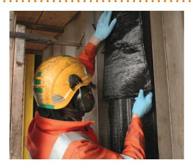
Our Technowrap SRS™ (Structural Rehabilitation System) utilises the unique features of carbon fibre technology intended for structural strengthening applications. It is less than one-quarter the weight of steel, which makes it 4 times as stiff on a weight to weight basis. It is approximately twice as strong in tension and it has a better fatigue performance than steel, aluminium or titanium.
